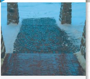
Apply Entry using a fan spray at a rate of 3/4 gallon per thousand.
